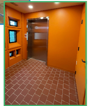
Top: A view of the new public elevator vestibule under construction.
